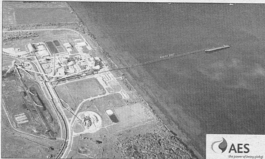
A rendering of AES Somerset's proposed lake-unloading facility depicts a 3,200-foot-long pier, where ships would dock to unload materials such as coal and limestone.
